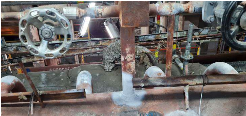
Fig.6. Example of cleaning preparation for MT testing of S – veldolet
